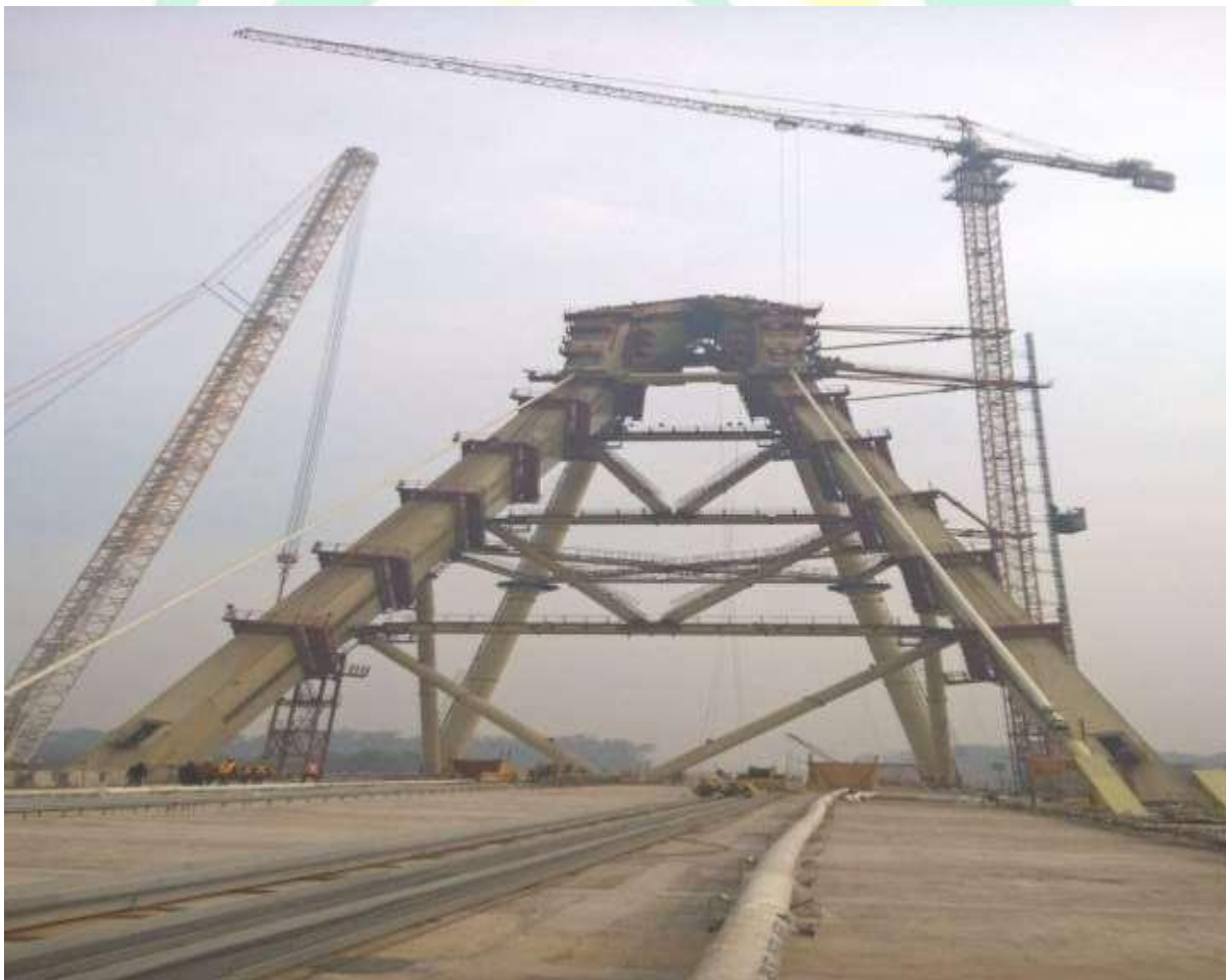
SIGNATURE BRIDGE, DELHI
