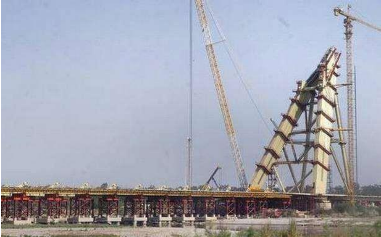
SIGNATURE BRIDGE, DELHI
