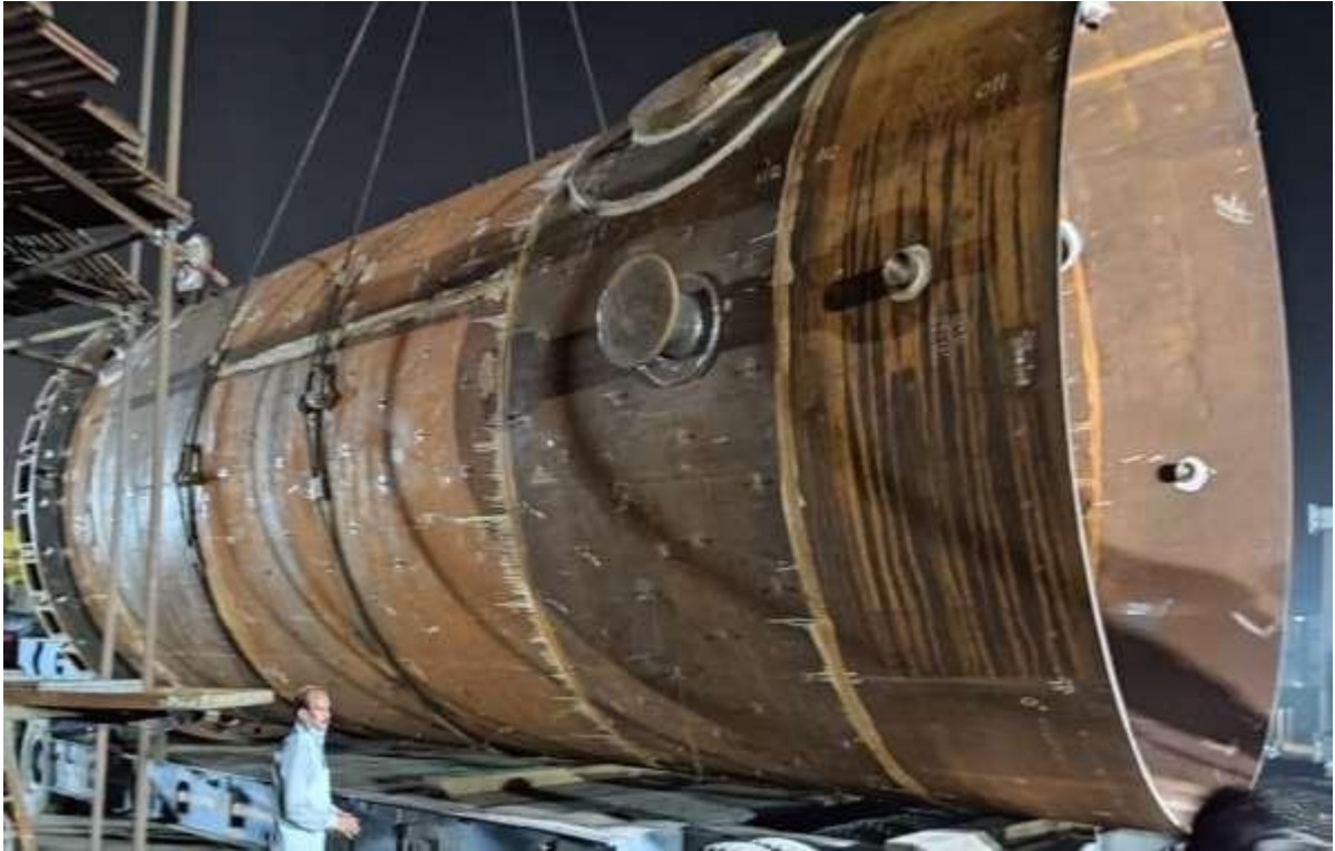
HRRL – SKIRT: HPCL – RAJASTHAN
