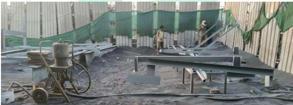
Blasting & Priming Area
